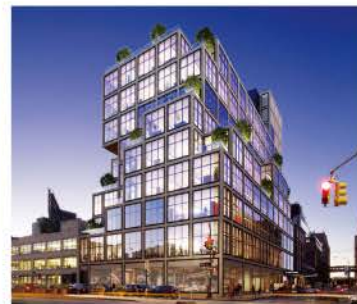
Mixed-use Building New York, USA
