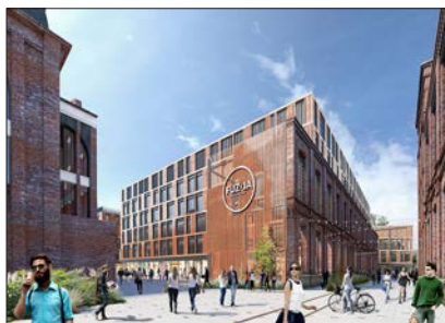
Fuzja Office is built on a former industrial site in the immediate vicinity of the Karol Scheibler textile factory and offers 22,000 sqm of rental space.
